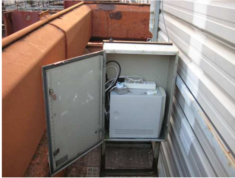
Figure 5: Gateway pc inside a box
