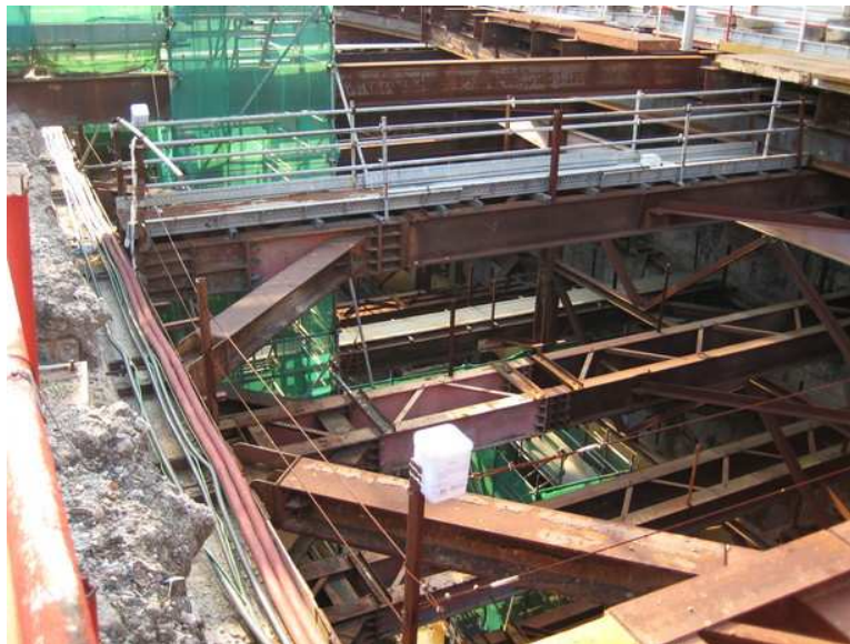
Figure 1: Construction site at Pasir Panjang MRT station
